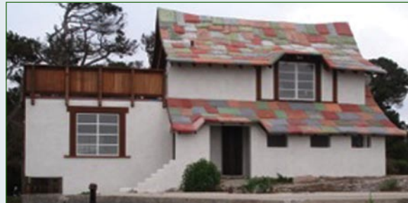
"After" the new exterior. Interior work is still needed.
