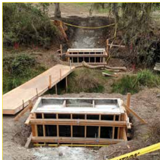
The abutments for the over crossing affectionately known as "Bart's Bridge" being installed after the winter saturated ground dried enough to be workable. Photo by Bart Bruno
